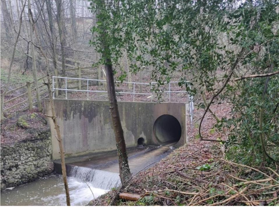
Photograph A3: Culvert Under A55
